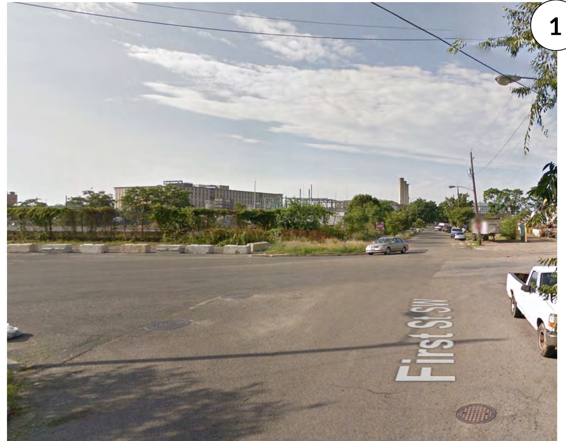
VIEW LOOKING SOUTH ON FIRST STREET AT THE INTERSECTION OF R STREET AND POTOMAC AVE SW
